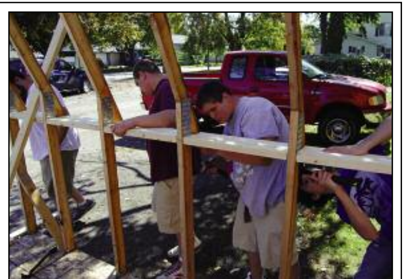
JOSH VALLENDER (from left), Austin Baker, Lucas Baker and Zach McLachlan were among the work crew members who recently assisted Cass City's Nick Karwowski, 18, with construction of a storage shed for the Living Word Worship Center in town. The project was the final requirement in Karwowski's climb to earn the highest rank in the Boy Scouts — the Eagle. (See story, page 8)
