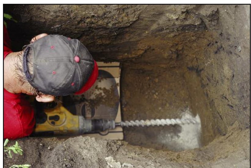
DRILLING A NEW water line from the new well into a local area house is Adam Tippets, an employee at F. E. Franzel Well Drilling LLC. The company recently was called to drill a new well after the owner's previous one dried up.
