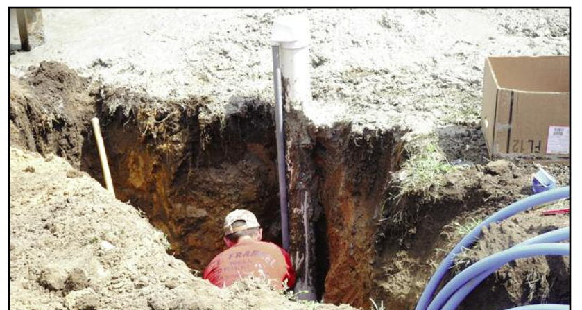
THE NEW CASING , which went 140 feet underground, is being worked on by Adam Tippets. The new casing is 5 inches in diameter and with the new electric 1/2 horsepower pump, it will be capable of producing 1,000 gallons of water for home use per hour.
