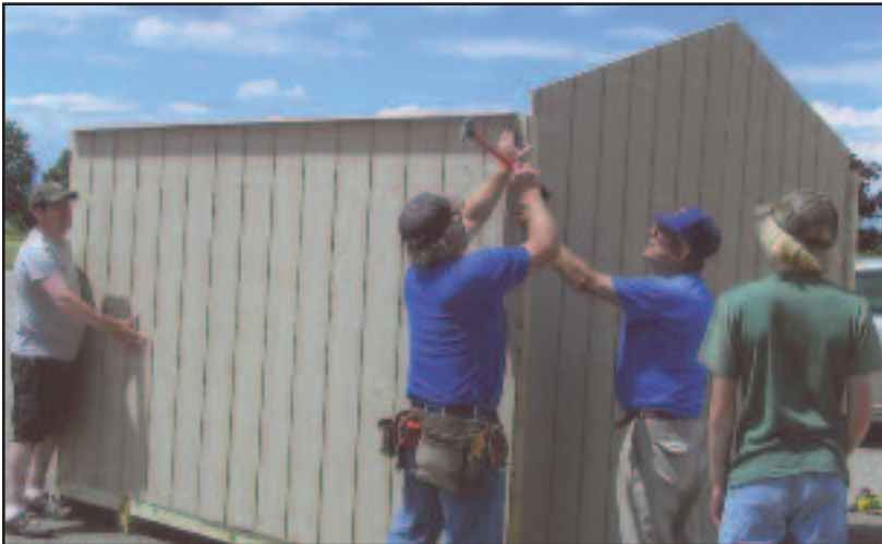
RON KITTLE (from left), Jim Albrecht, Bob Wood and Travis Albrecht all volunteered to join Jacob Kittle's Eagle Scout Project "work crew".
