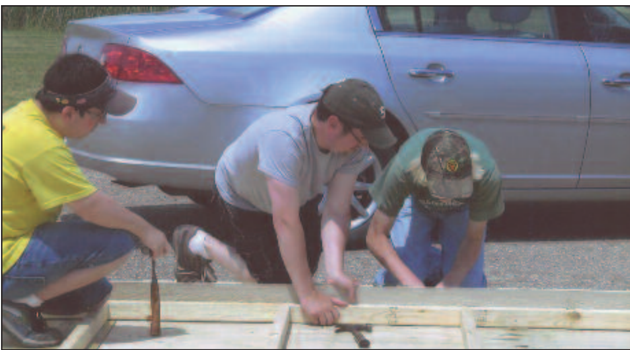
CASS CITY HIGH School senior Jacob Kittle (from left), his dad, Ron Kittle, and Travis Albrecht construct a section of the storage unit built for the Cass City United Methodist Church in July. Completion of the project was Jacob's final step in becoming an Eagle Scout — the highest rank in Boy Scouting. Kittle is a member of Boy Scout Troop 594, Cass City.
