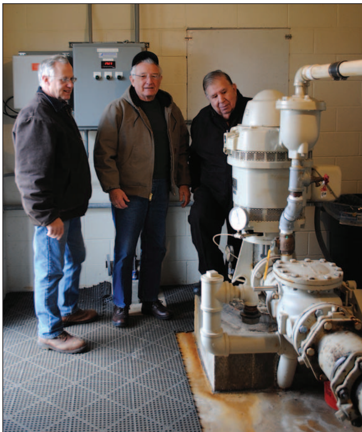
VILLAGE OFFICIALS, from left, Gary Barnes, Carl Palmateer and Peter Cristiano examine Cass City's number 3 well. Repairs to the well's pump is the focus of a special meeting Wednesday.
