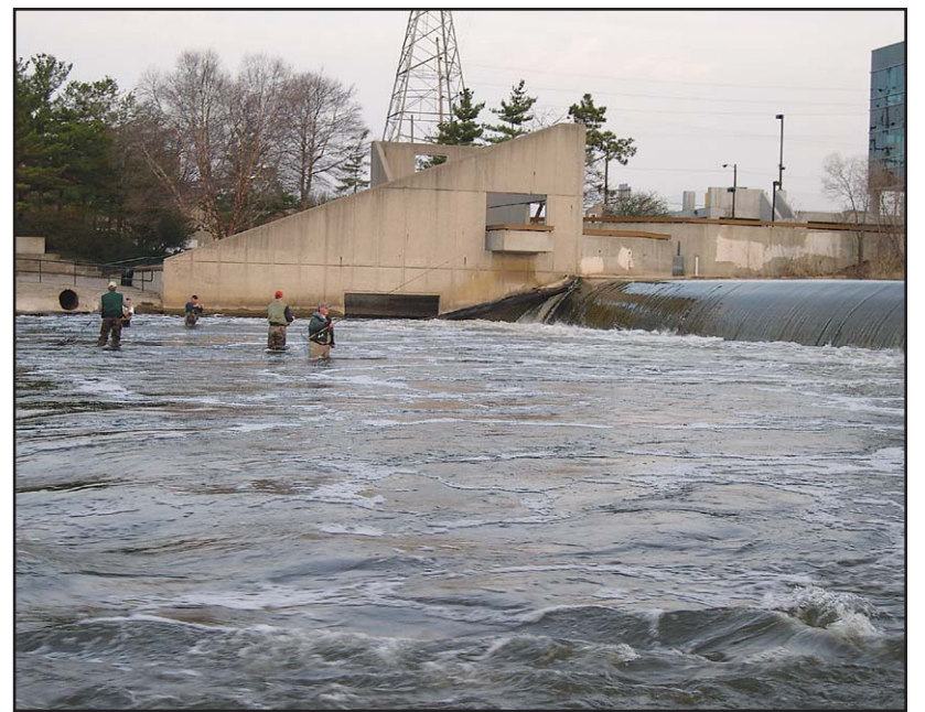
FISHERMEN in Grand Rapids cast for steelhead below the Sixth Street Dam. In the background is the city's fish ladder, where visitors can watch steelhead and other fish make their way past the dam via a series of concrete steps.
