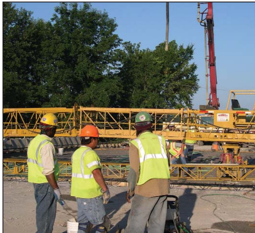
WORKERS WITH J. Slagter & Son Construction, Wayland, replaced about 2 inches of concrete - roughly 30 yards in all — on the deck of the Cass River bridge east of Cass City Thursday morning. The $180,000 maintenance project, slated to be completed by early September, includes replacing the guardrails, and replacing the concrete and asphalt approaches to the bridge in order to provide motorists with a smoother ride, according to Michigan Department of Transportation officials.
