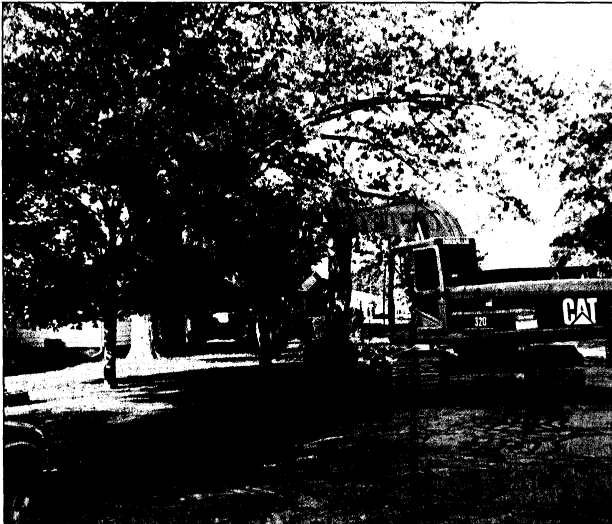
WORK TO REPAIR a collapsed storm sewer along Church Street began Monday in Cass City. Village officials are hoping for sunny skies over the next 2 weeks to minimize their costs.
