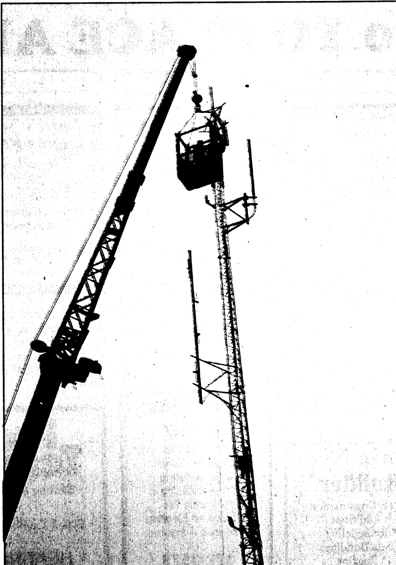
TALL ORDER - TotalCom employees repair antennas damaged by lightning on their tower in Cass City last week. The work required them to be lifted by a crane to a height of some 186 feet.
