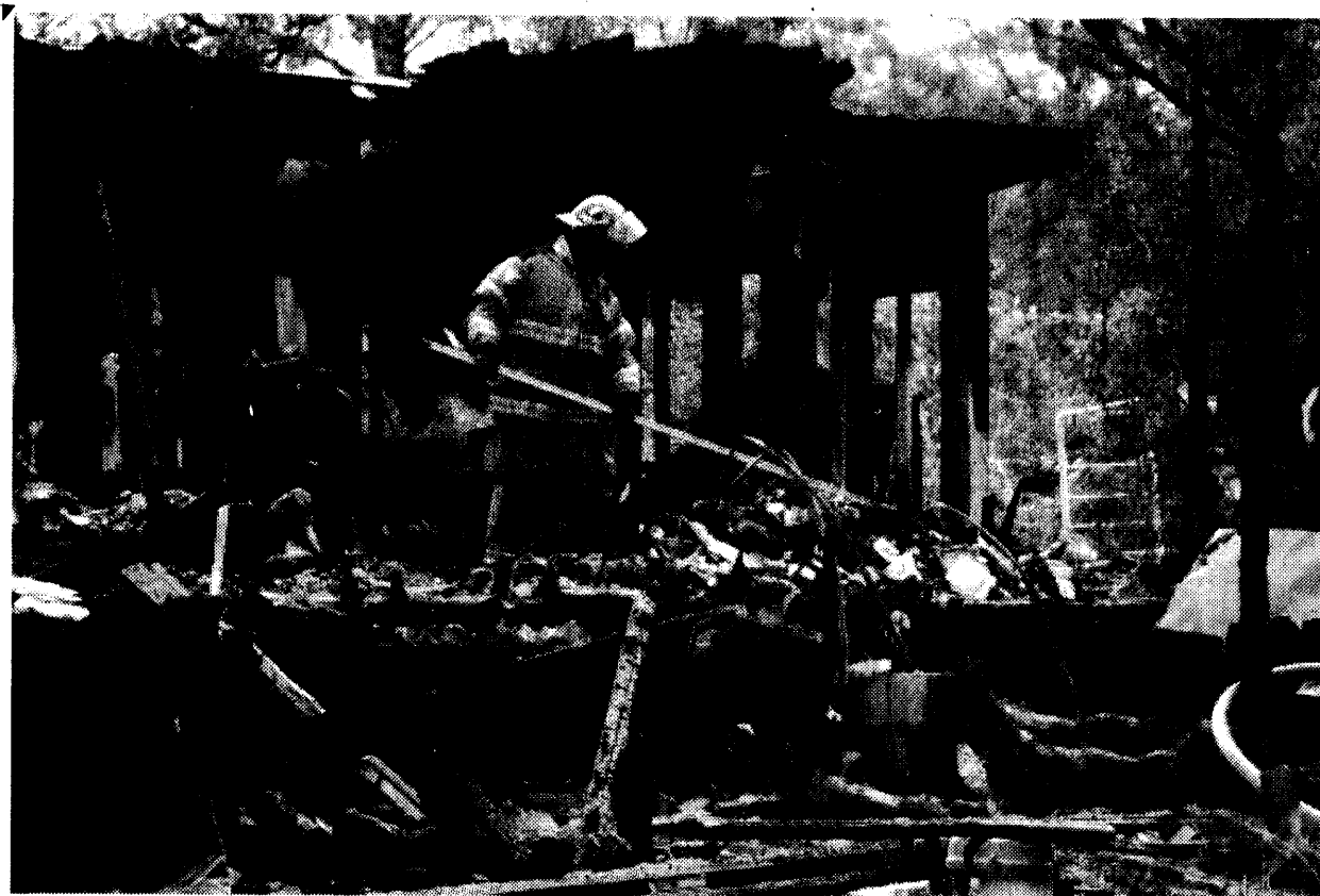
A FEW support beams remain standing after a house fire at 6796 Severance Road the afternoon of July 11. Six fire departments worked 3 hours to put out the fire, which caused an estimated $90,000 of damage.
