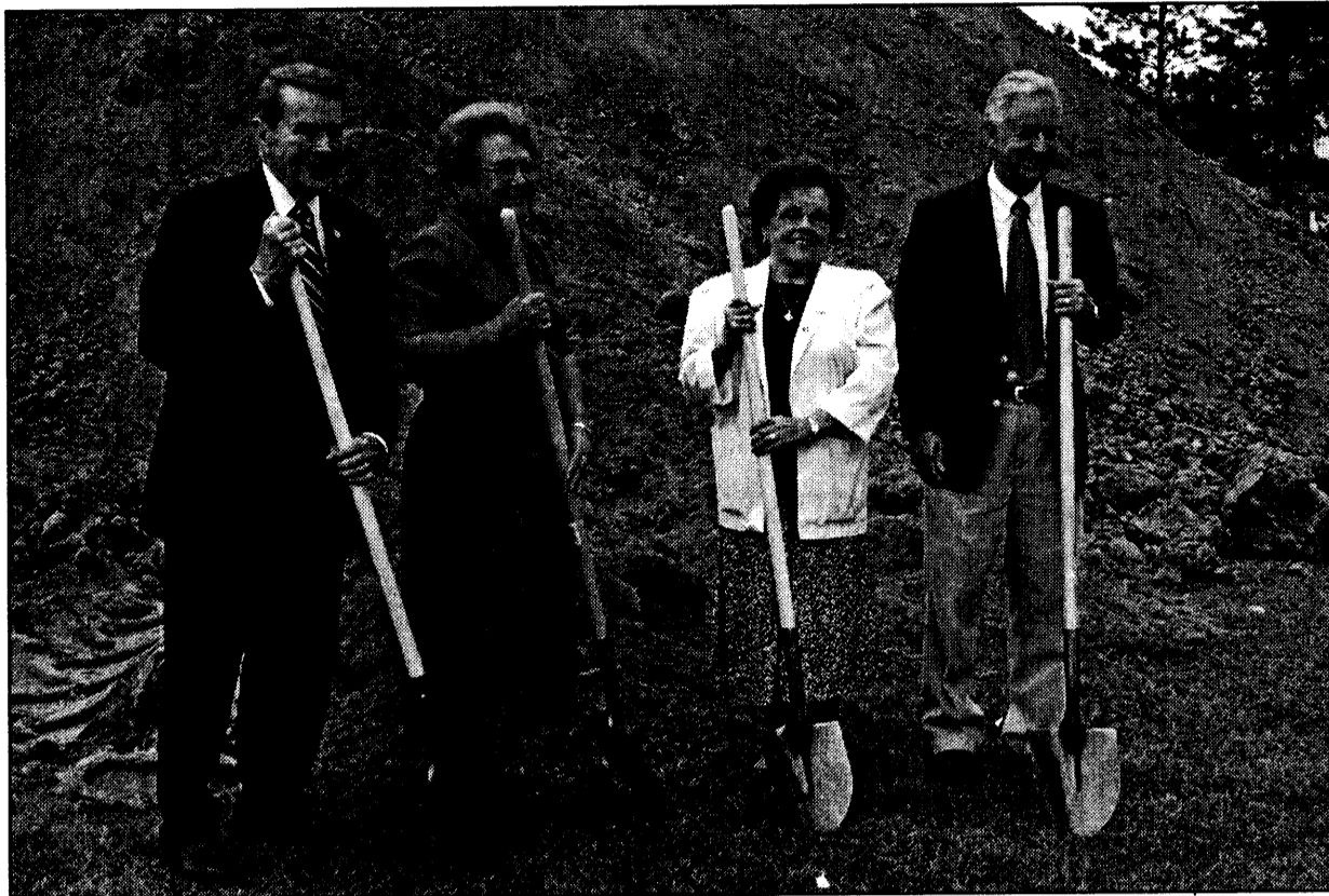
BREAKING GROUND for the "Generations - The Mary Ann Vandemark Center" Friday were (from left) Congressman Dale Kildee, Mary Ann Vandemark, HDC Board Chairperson Della Hammond and Michigan USDA Rural Development Director Gene DeRossett.
