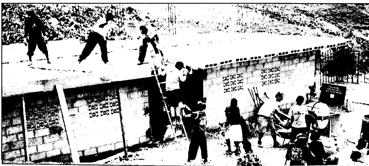
MEMBERS OF THE mission team work hand in hand pouring cement at the Alison Emmert Education Wing, using only 5-gallon buckets and a single cement mixer powered by a generator.
