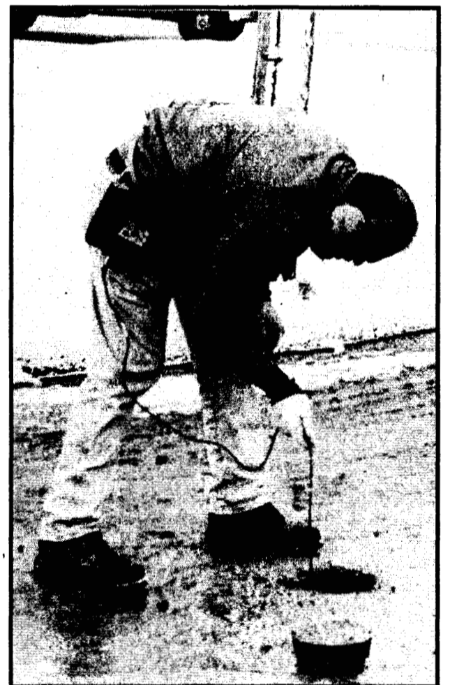
LEAK buster - Scott Wilson from Aqua-Line "listens" for water leaks in a water main valve at the corner of Main and Ale streets Monday morning.
