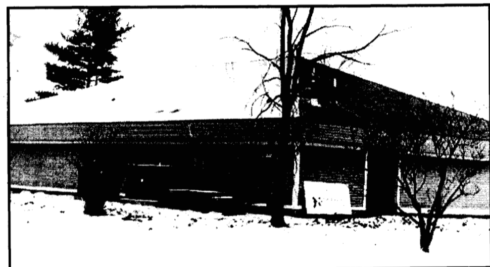
NEW CONSTRUCTION in the Downtown Development Authority area such as this dialysis center generates dollars for DDA.
