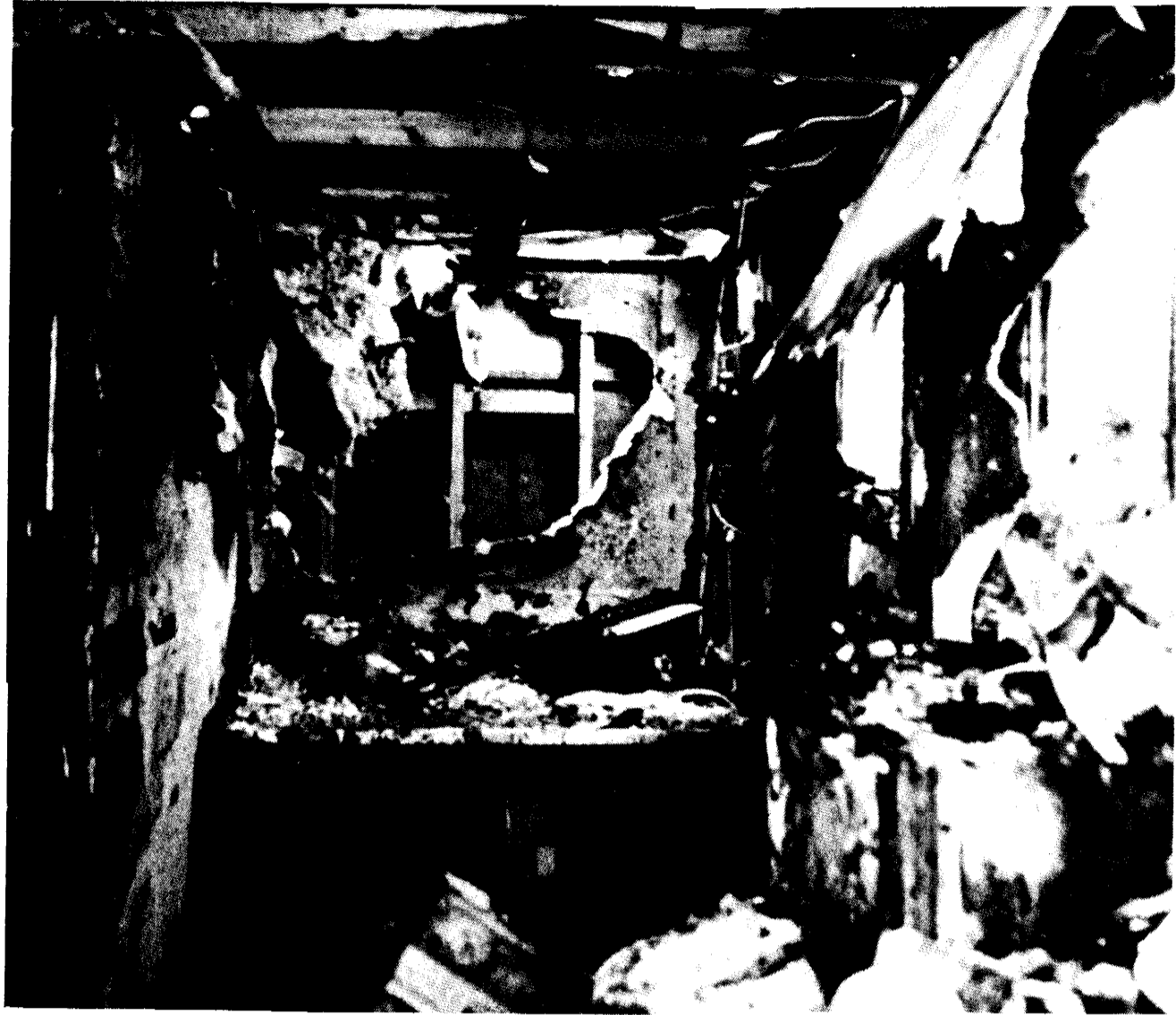
A GAS LEAK from the stove (pictured on right) caused an estimated $40,000 in fire damage Tuesday at the residence of Lee and Theresa Strickland of Gageton.
