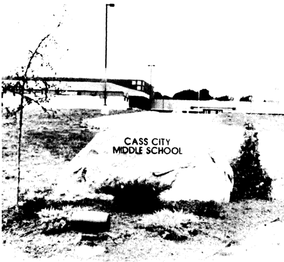
FINISHING TOUCH — Doerr Landscaping, Cass City, recently dressed up the entrance to the new Cass City Middle School, where students will soon be welcomed back for the start of the 1998-99 school year.
