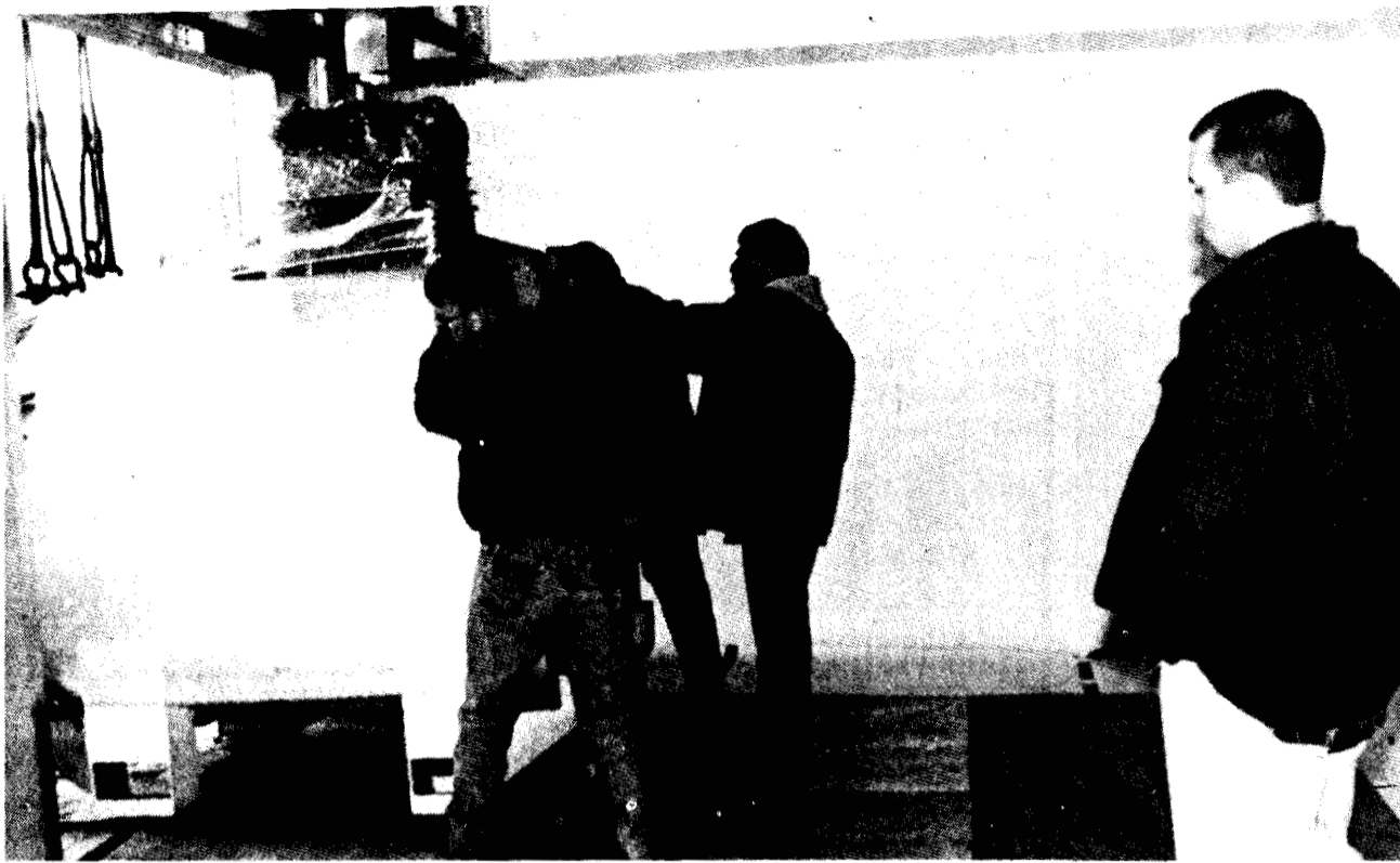
MIGHTY MAGNET — A magnet some 30,000 times stronger than the magnetic force of the Earth, used in Magnetic Resonance Imaging (MRI), was delivered Friday to the new Thumb MRI Center. Above, workers position the magnet inside the MRI room at the Cass City area facility, which is slated to open for business in just a few weeks.
