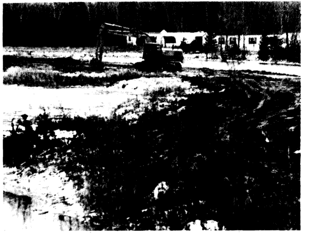
AFTER MONTHS OF waiting, a Cass City businessman has received permission from the DNR to develop a portion of this wetlands, located at the south end of Doerr Road, into modular home sites.
