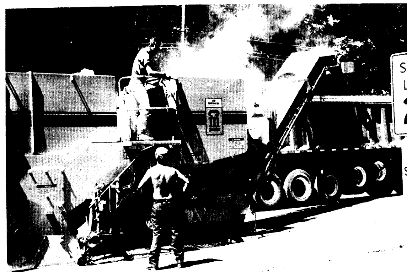
CONSTRUCTION WORKERS began removing the asphalt on Seeger Street Wednesday. A one mile stretch of the street is to be torn up and re-asphalted. Additional curbs and handicap ramps for sidewalks are also planned.
