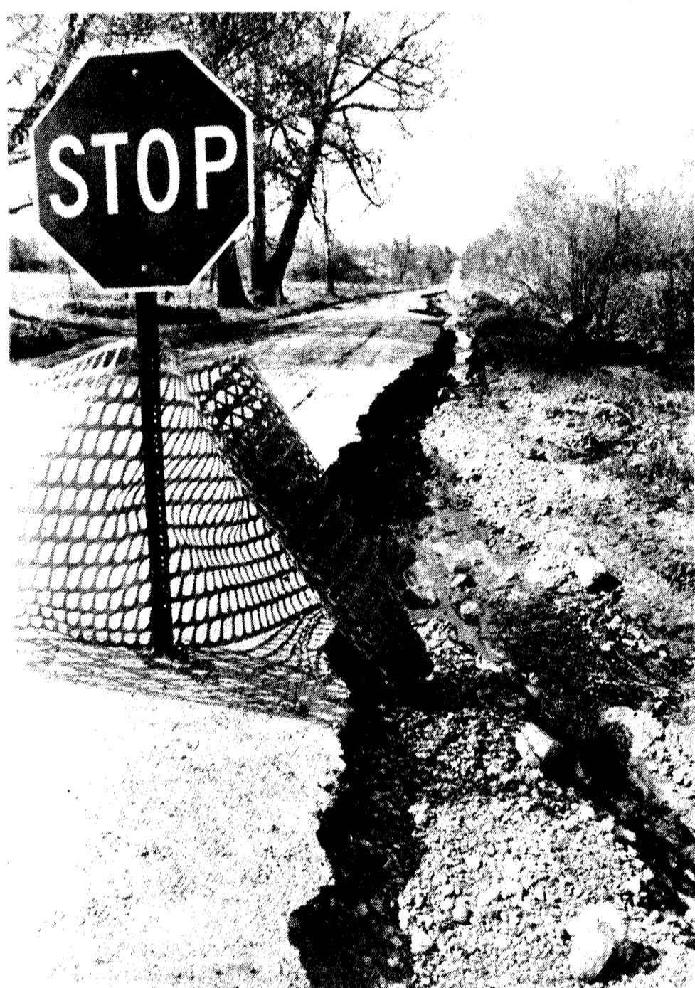
MOTHER NATURE overwhelmed the Thumb with rain in 1996. June flooding resulted in a Presidential Disaster Declaration in several counties, including Tuscola, which has received $3.26 million in federal/state grants and loans to repair homes, businesses, roads and drains.
