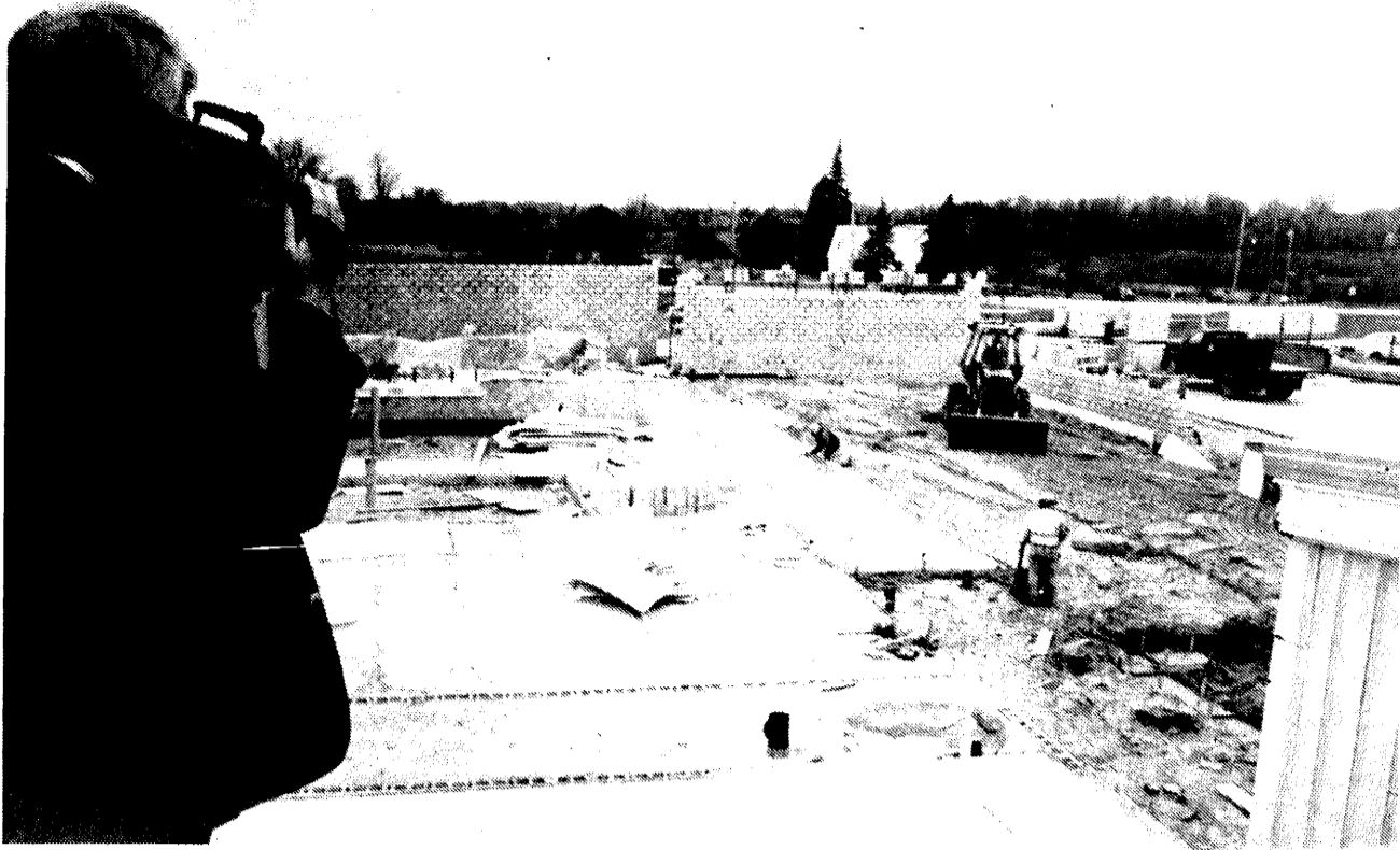
NEW CLASSROOMS ARE beginning to take shape at Kingston High School, where work on a 13,000-square-foot expansion project has been underway since October. Above, school Supt. George Goodchild videotapes the progress from the rooftop.
