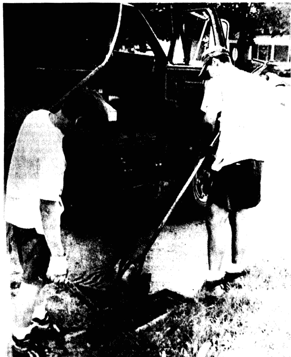
SOMEBODY'S GOT to do it. Cass City DPW employees Jason Mohr (left) and Al Prosowski recently had the unenviable task of cleaning out the village's more than 400 storm sewer catch basins. The annual maintenance chore takes about 2 weeks to complete, according to Village Manager Lou S. LaPonsie.
