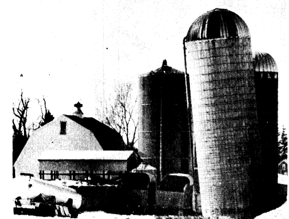
LEANING TOWER of grain — Deterioration at the base of an old silo at Laurie Farms northwest of Cass City caused the structure to begin a slow but certain descent to the ground about 2 weeks ago. The silo contains 10,000 to 15,000 bushels of corn, according to Doug Laurie, who said a professional demolition crew will be in this week to bring the structure down safely.
