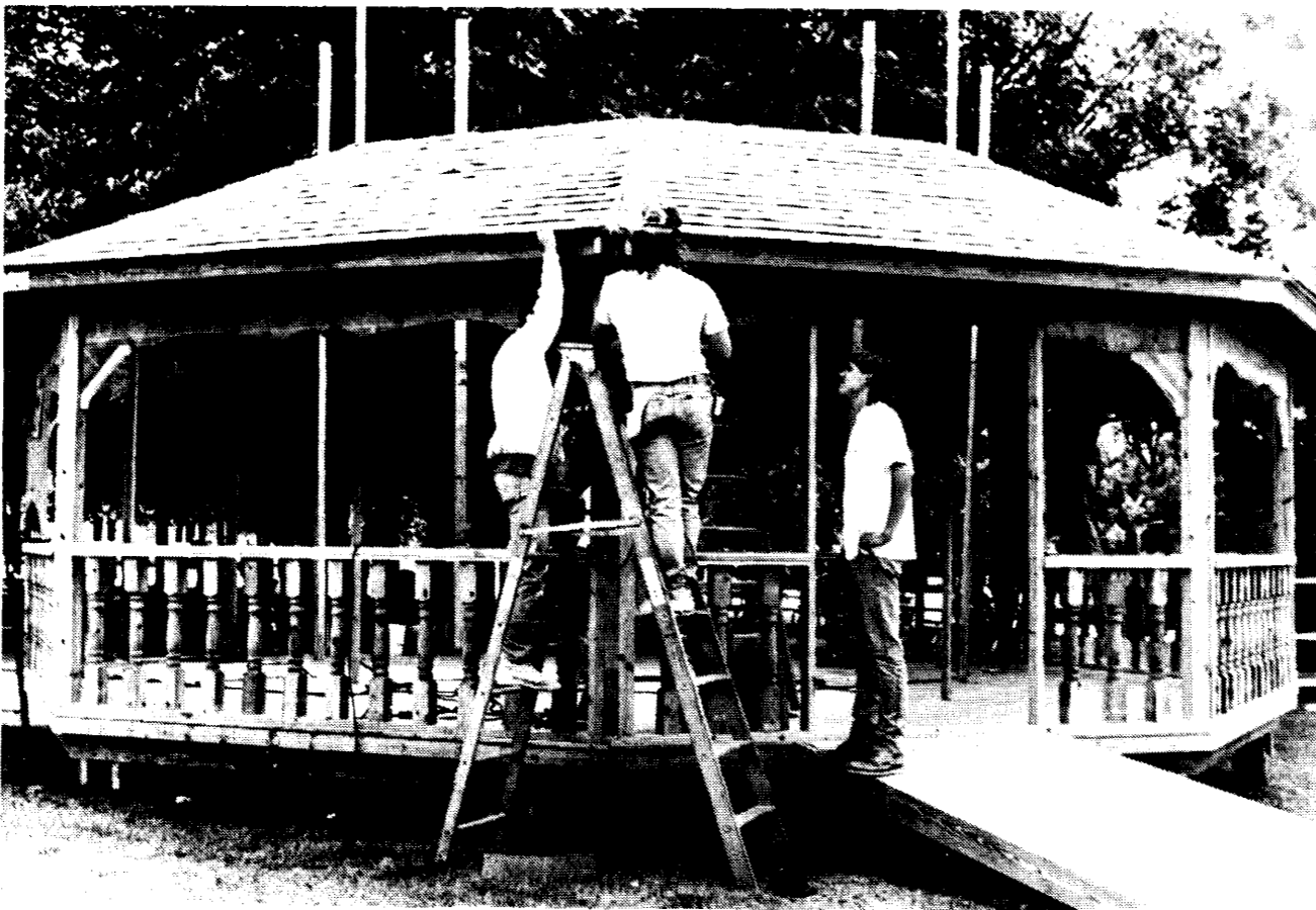
A CREW FROM Joe's Tables, Pinconning, quickly assembled the Cass City Lions Club gazebo near the corner of Church and Ale streets in Cass City Monday, in time for the village's annual July 4 Festival. Work on the $11,000 structure, which is being donated to the village, was delayed by last week's rain.
