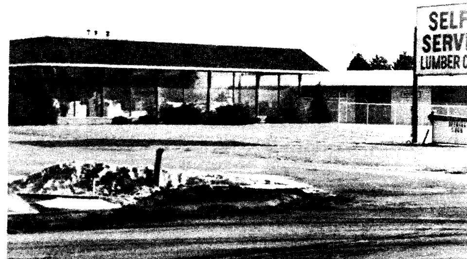
MOVING INTO THE vacant auto dealership this week was Self Serve Lumber Co. It's an indication of the healthy condition of the building and supply business in the community.
