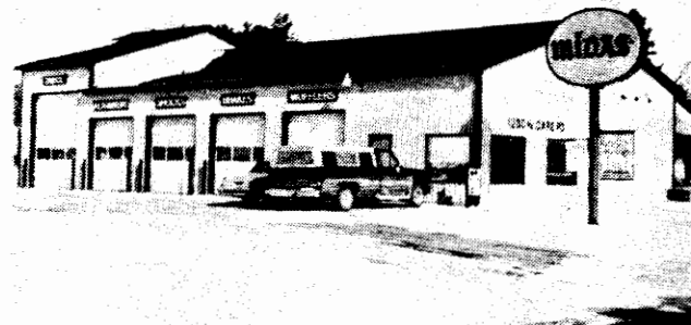
MIDAS MUFFLER is moving into its second year of business in its new facility on West Caro Road.
