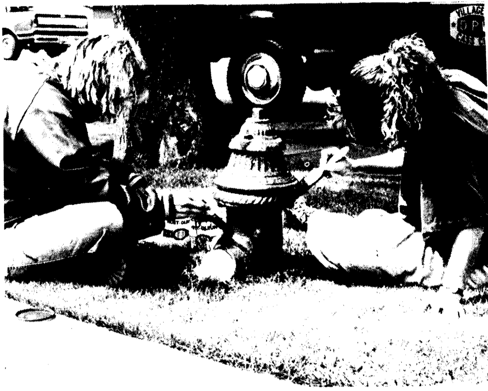
THE VILLAGE OF Cass City sent out employees Jodi and Jandi Hillaker to give the town's fire hydrants a new coat of paint last week.
