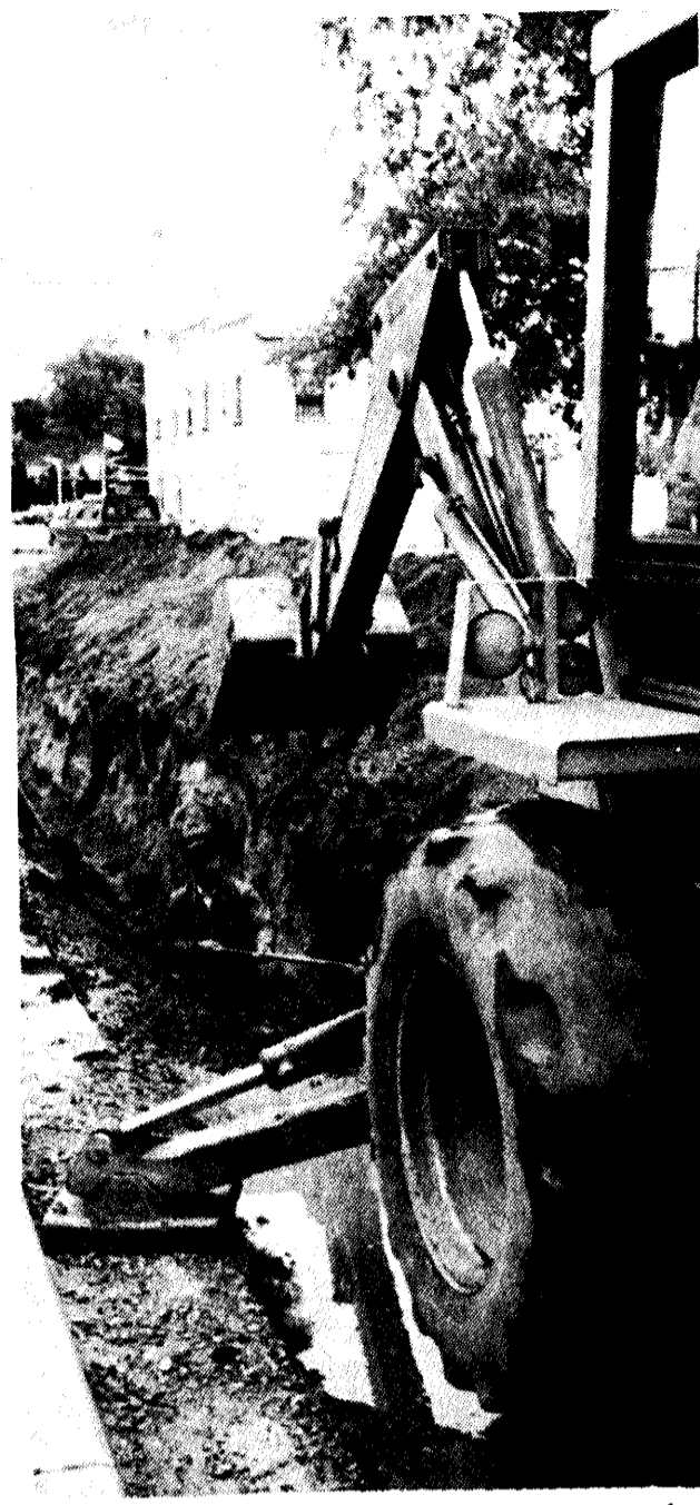
CASS CITY DPW workers have been busy replacing a water main along South Alley and Oak Street. Part of an on-going maintenance program in the village, this year's projects replaced 1,600 feet of main at a cost of $48,000.
