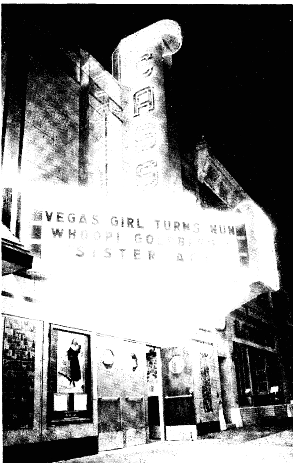
THE CASS THEATRE has retained its small town appearance and flavor over the years, but today's features are shown on state of the art projection equipment.
