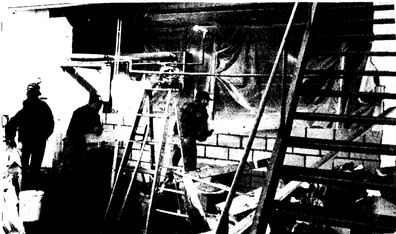
REPAIRS ARE BUSILY being made at Sommers Bakery in Cass City, where a gas explosion rocked the Main Street building last week, injuring a pair of bakers and causing extensive structural damage. Replacing the rear wall of the bakery Monday were (above, left to right) Les Kendall, Mark Tuckey and Alvin McKee, all of Tuckey Builders, Cass City.
