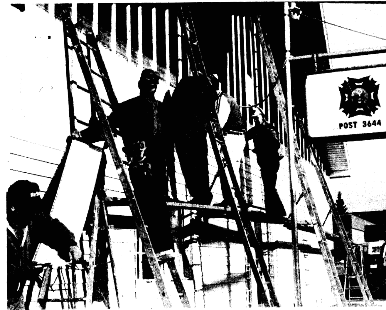
TEAM WORK — CASS City VFW members took advantage of beautiful weather Friday morning to install siding on the front of their new post hall west of Weaver Street. Sharing the workload above were (left to right) Dean Fulcher, Emerson Kennedy, Harold Blehm, John Zawilinski, Dick Haney and Hazen Guinther (not pictured)
