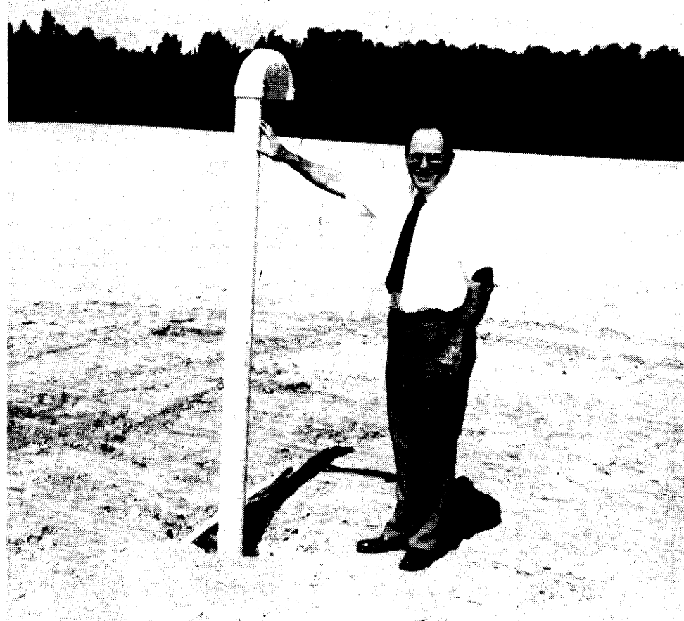
CASS CITY'S LANDFILL looks more like a sand dune than a dump following several weeks of work tied to the village's $334,000 landfill closure project, which is expected to be completed this fall. Above, village Manager Lou S. LaPonsie stands next to one of 4 gas vents installed on top of the Type II site.
