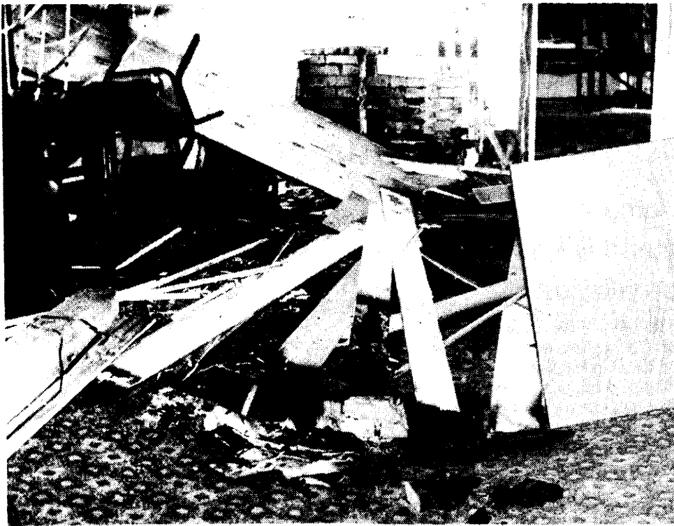
THE FIRE WIPED out floor joists in the central portion of the inn, burning a hole through the floor of a game room and causing the floor to bow (above).
