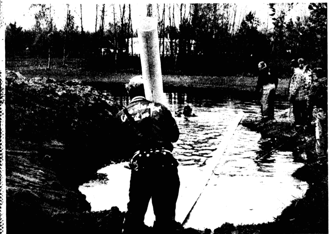
CARO FIREMAN GARY Corkins steadies the 6-inch PVC piping used to make a dry hydrant in a pond just south of Deford Saturday morning. After Tuscola County Dive Rescue Team Capt. Duane Sprague (above, in the water) helped set the piping in place under water, the trench was filled back up with sand.
