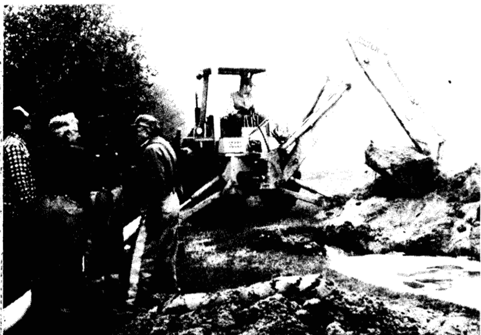
ELKLAND TOWNSHIP Fireman Randy Middleton digs a trench in preparation for the installation of a dry hydrant at the Clinton Warner residence. Standing by are (from left) Elkland Township fireman Roger Hurley, Caro fireman Dick Damm, Elkland Fire Capt. Milt Connolly and Chief Dick Root.
