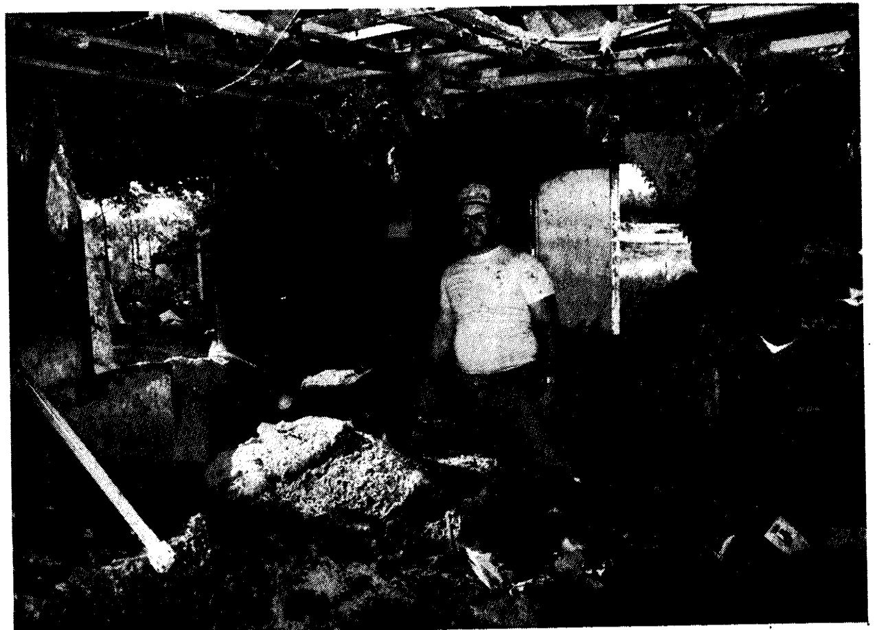
DESPITE A HIGH number of home fires this year, including a blaze in June that gutted the Floyd Morrish residence (above), area fire fighters reported no fatalities and only minor injuries.
