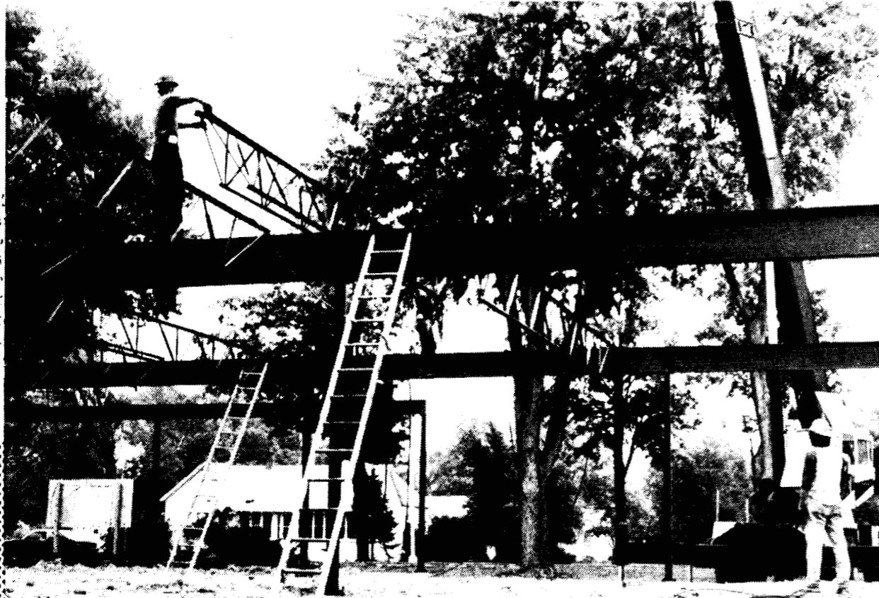
PROGRESS — SANILAC Steel Inc. workers last week constructed the frame that will support the new Jordan College building in Cass City. The Thumb campus is slated to open in early January for the start of the winter semester.
