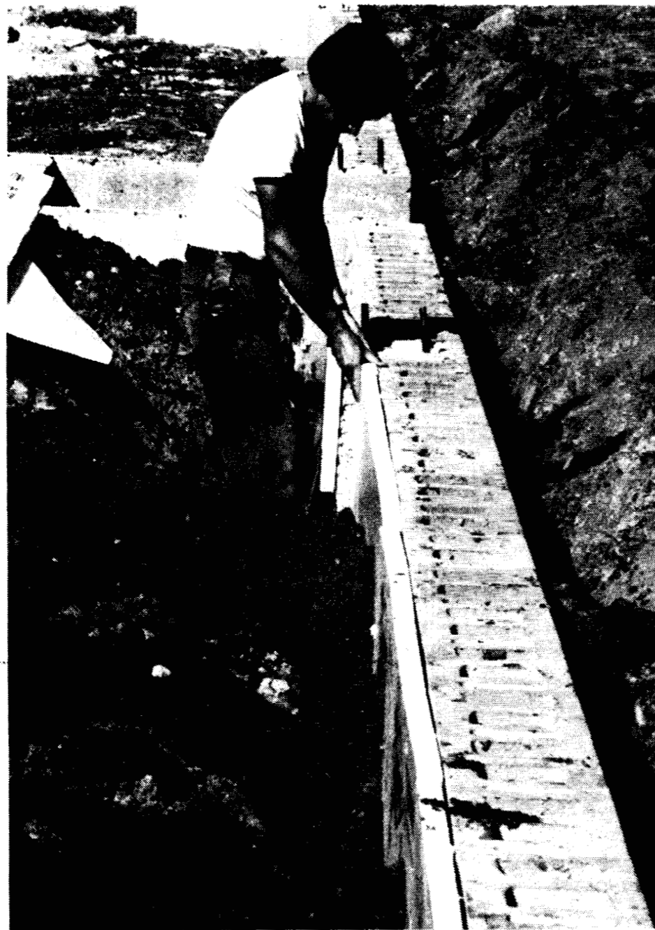
HERRON BUILDERS crew member Carl Russell, Cass City, places insulation along the floor base of the college building a few days before Sanilac Steel Inc. arrived at the construction site.
