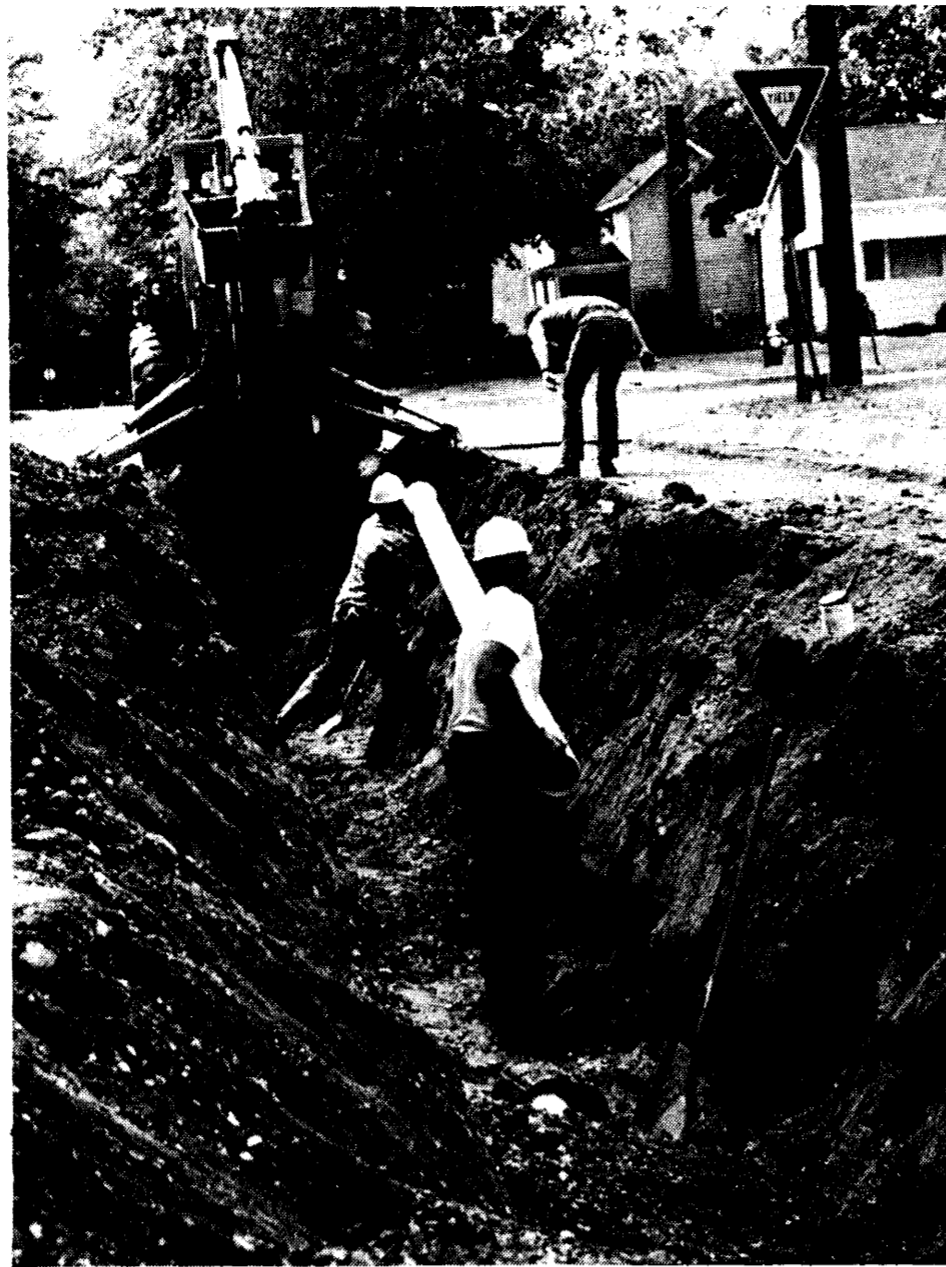
REPLACEMENT OF AN old 4-inch water main with a 6-inch plastic main along Third Street, from Ale Street to Woodland Avenue, is expected to be completed by the end of this week. Village officials hope the project will clear up problems with rust in Third Street residents' water.
