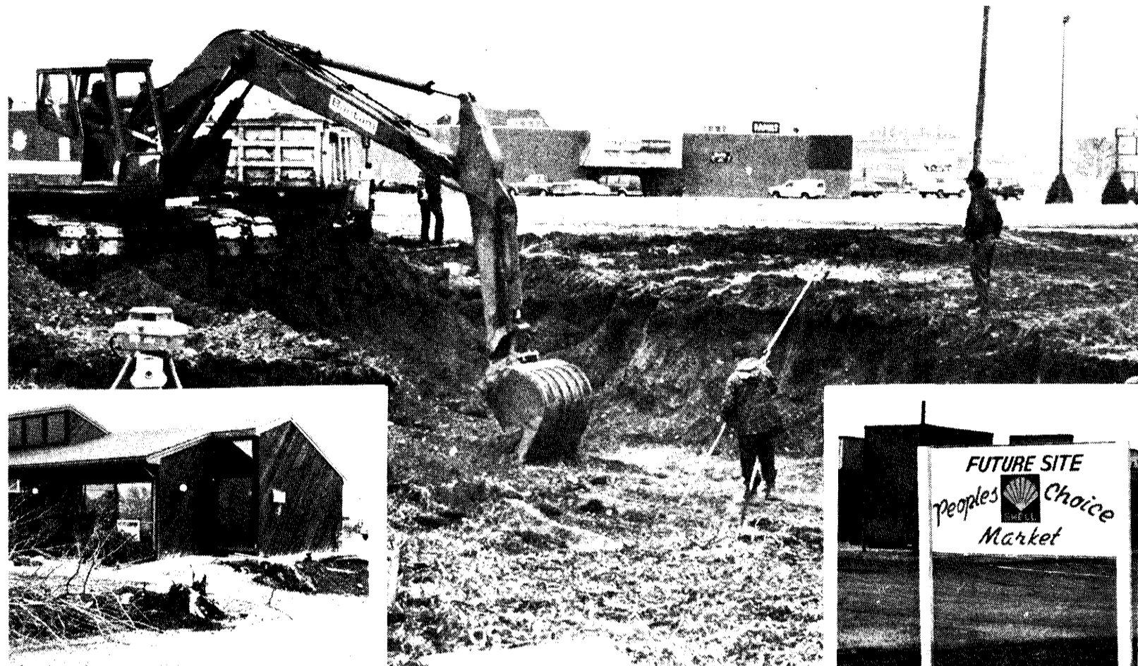
PREPARATIONS FOR THE planned relocation of an office complex (inset, left) south of its present location near the M-81-Doerr Road intersection are well underway. Above, workers dig a new foundation for the complex, which will be replaced by a combination convenience store and gas station, brought to Cass City by People's Oil and Gas Co., Pigeon.
