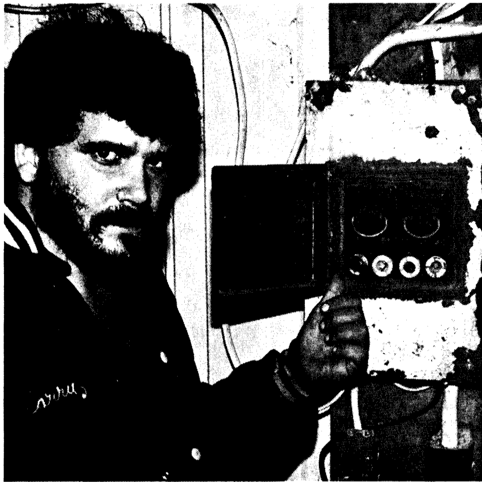
LARRY BUEHRLY POINTS to the burned-out casing of a fuse in his pole barn, which along with his house is only a few yards from where the lightning struck Friday. The fuse, Buehrly said, was blown out when the lightning made contact with an electrical line that runs into the barn and house. (See story, page 1).
