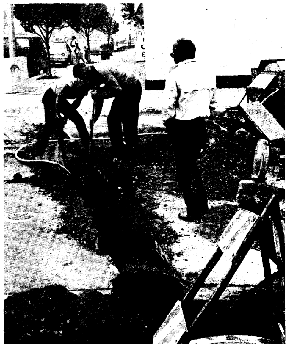
EMPLOYEES OF C & L Electric, a Lansing contractor, prepare to lay cable across Maple Street near Main Street for emergency flashers that will warn motorists of oncoming fire trucks and other emergency vehicles. Watching the work above is Rich Winiarski, a Michigan Department of Transportation construction inspector.
