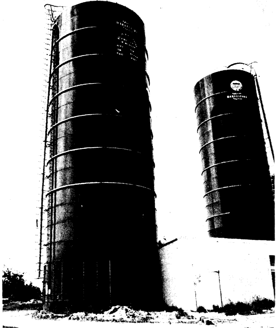
JIM AND PAUL WHEELER were the first farmers in Michigan to have a model "3189" Harvestore silo (left). The Snover farmers were less than satisfied with the structure, and last week were awarded $1.7 million in a lawsuit against A.O. Smith Harvestore Products, Inc., over milk and feed losses they attribute to the 3189.
