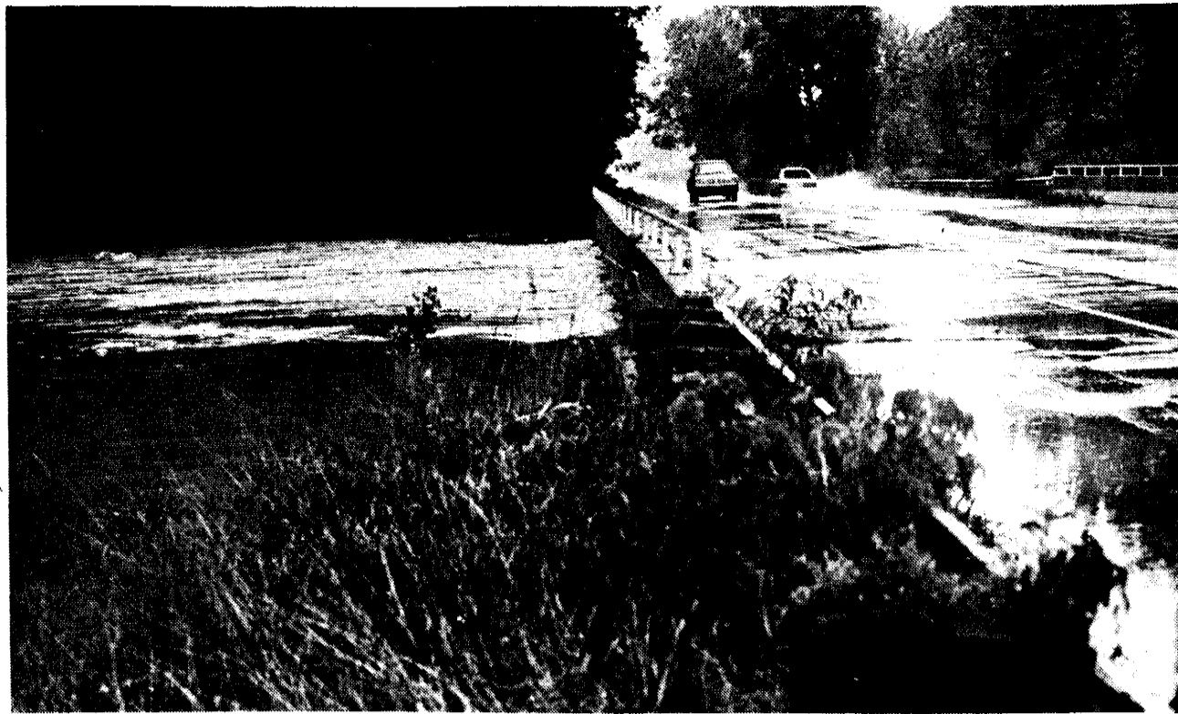
WATER CASCADING across the bridge on M-81 at the Cass River, east of Cass City, was repeated on bridges all across the Thumb.
