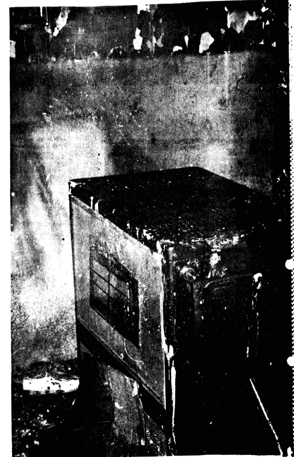
COMBUSTIBLE MATERIALS placed too close to this wood burning stove caused a fire in the Deford area that destroyed a two-story house.
