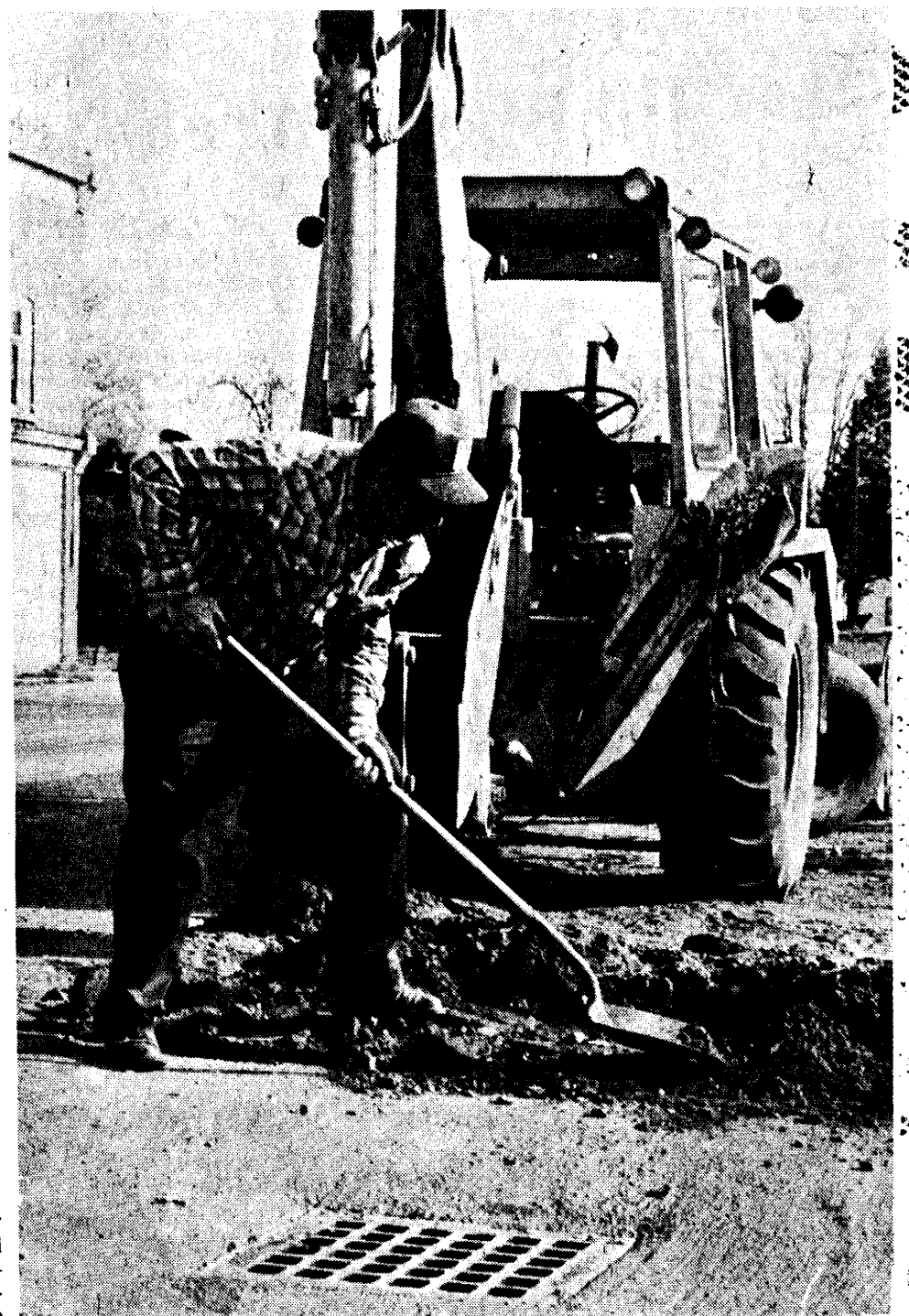
CONTRACTOR DICK LITTLE of Caro puts the finishing touches on a storm sewer catch basin in Deford. So far three new catch basins have been installed in the community.
