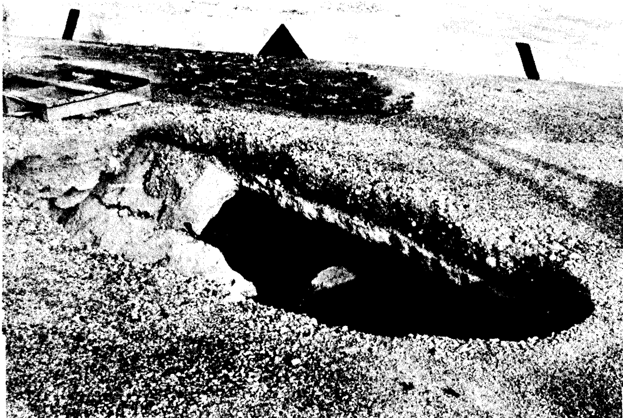
CAVE-IN - A 48-inch storm sewer south of the old Nestles Building recently caved in. The village estimates the cost to replace the sewer will be $15,500.
