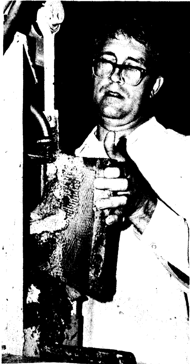
WITH A WATER heated vibrating knife Owen Pierce cuts the wax cap off a honeycomb frame.
