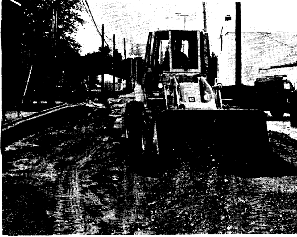
CITY CREWS were busy last week preparing the south alley, from West to Seeger Streets, for a new coat of asphalt. The alley is expected to be paved in early September.
