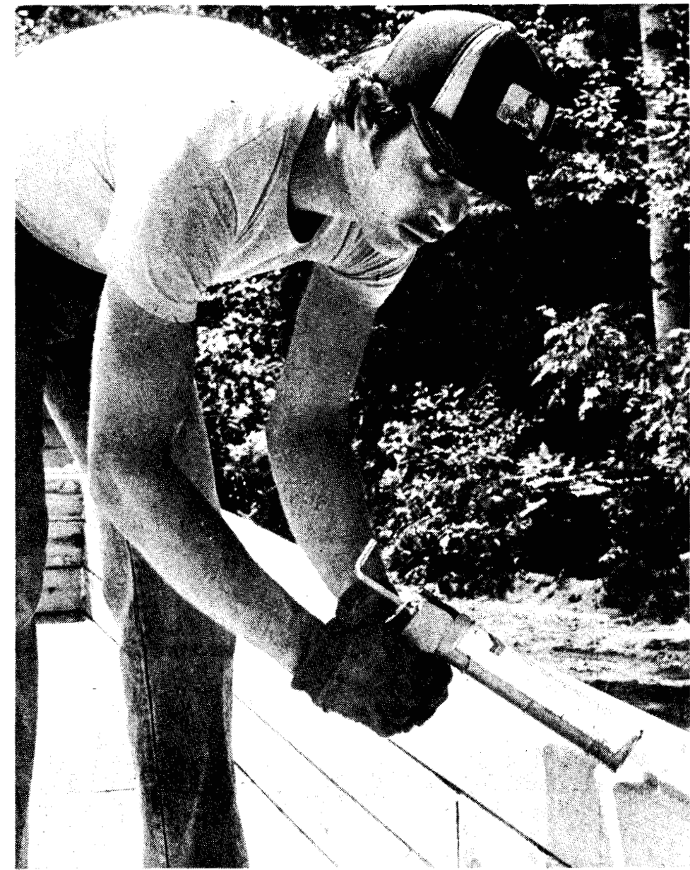
HELPING A FRIEND - Brian Crass liberally applies caulk between the logs of the Winchester home, to seal out air leaks.
