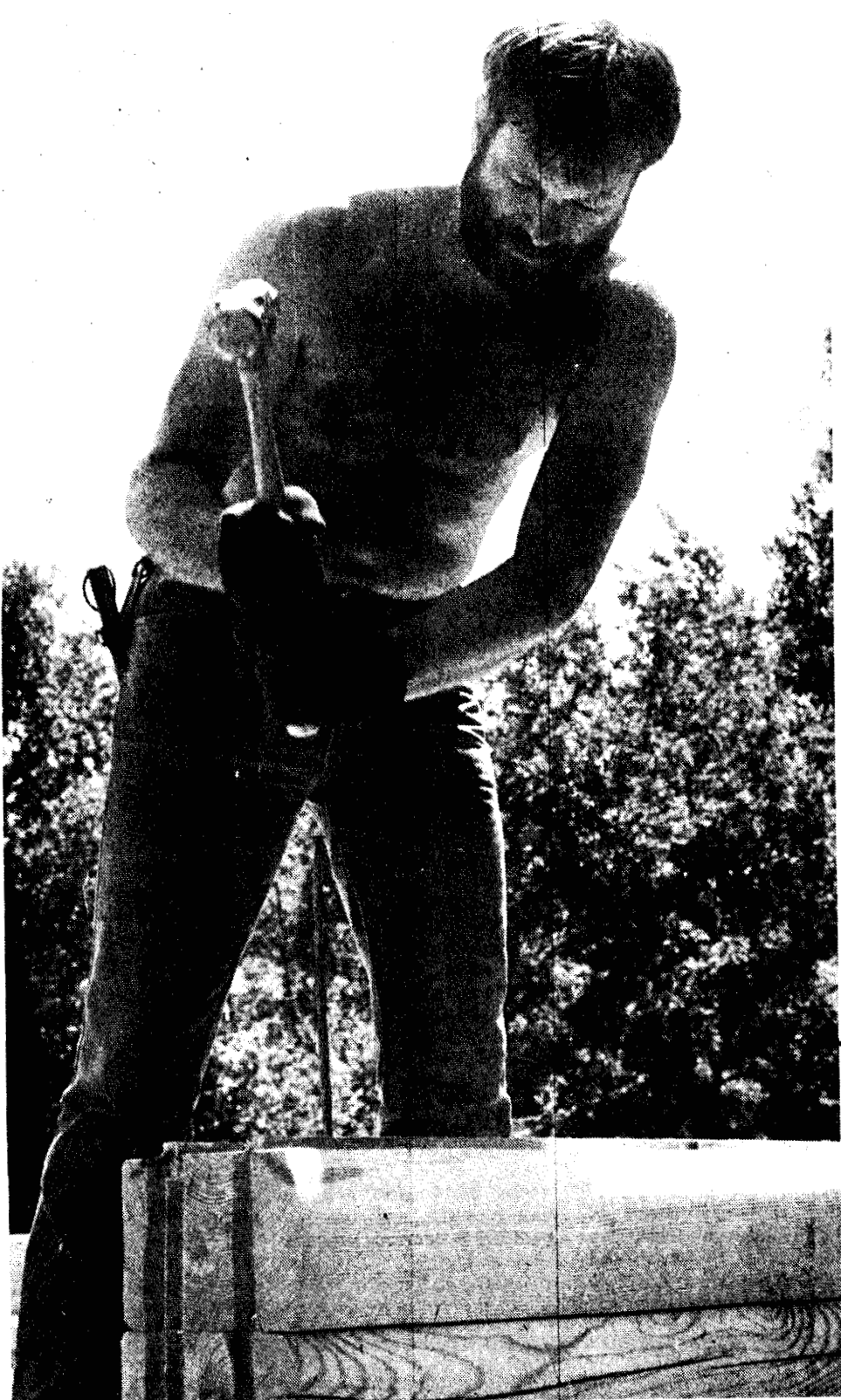
DAN WINCHESTER prepares to drive a 10-inch spiral nail into one of the logs of his new Dutcher Road log home.
