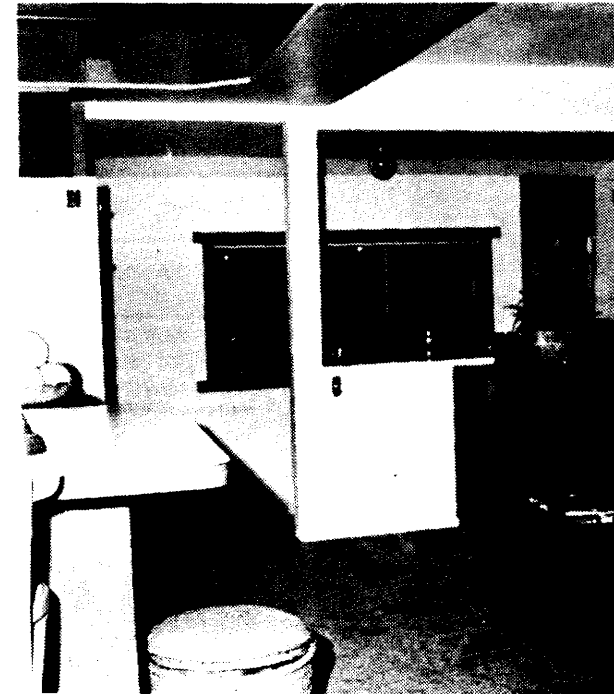
PART OF the restoration includes the windows on the north wall and new headers in the kitchen-dining room.
