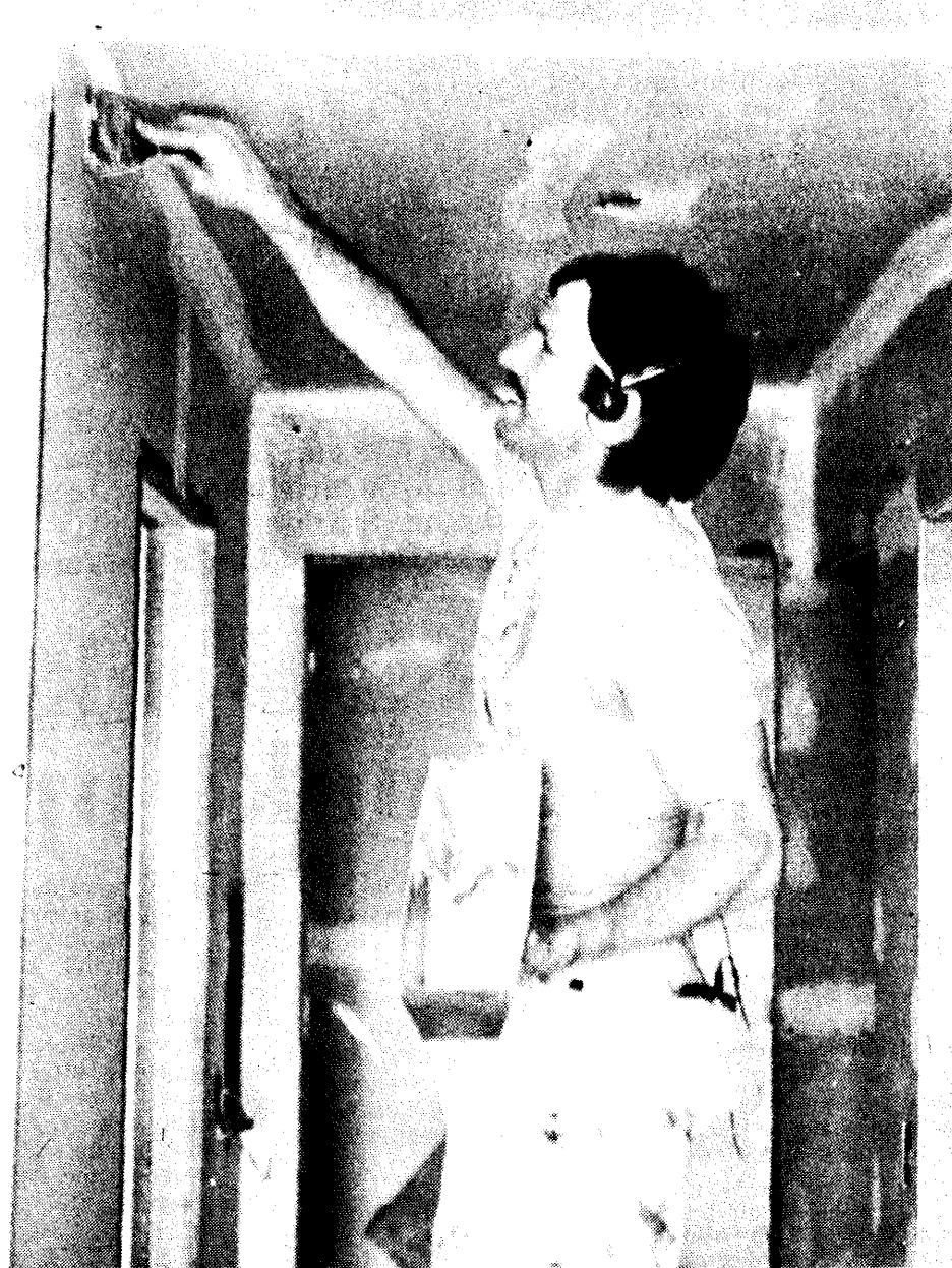
JOHN EBERHART puts the final touches on the interior walls at the new senior citizens apartment complex located on Woodland St., Cass City.
