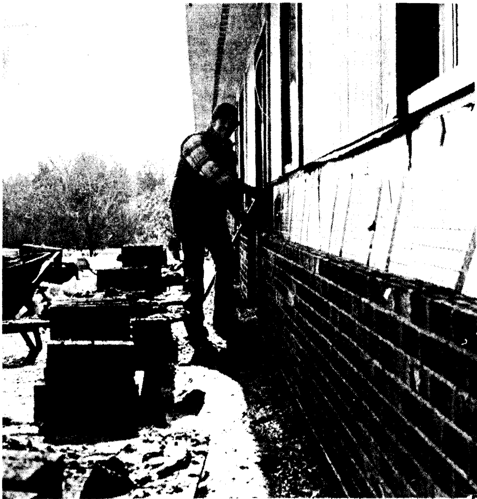
BRICK LAYER Gordon Smith, Cass City, an employee of Steve Putman Contracting, Caro, lays another row of bricks at the new senior citizen apartment complex.
