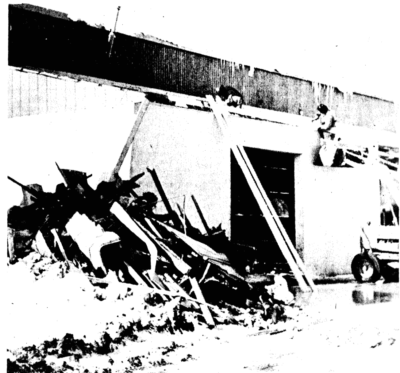
REPAIRS WERE ALREADY underway Tuesday at General Cable after snow caused the roof of a small addition to the main building to collapse.
