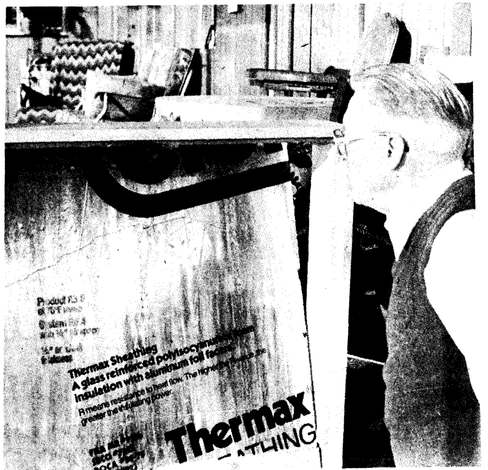
BY BLOWING on the door of an air damper that Severance designed and built, the door swings open. The damper prevents the heat from reverse circulation in the house.
