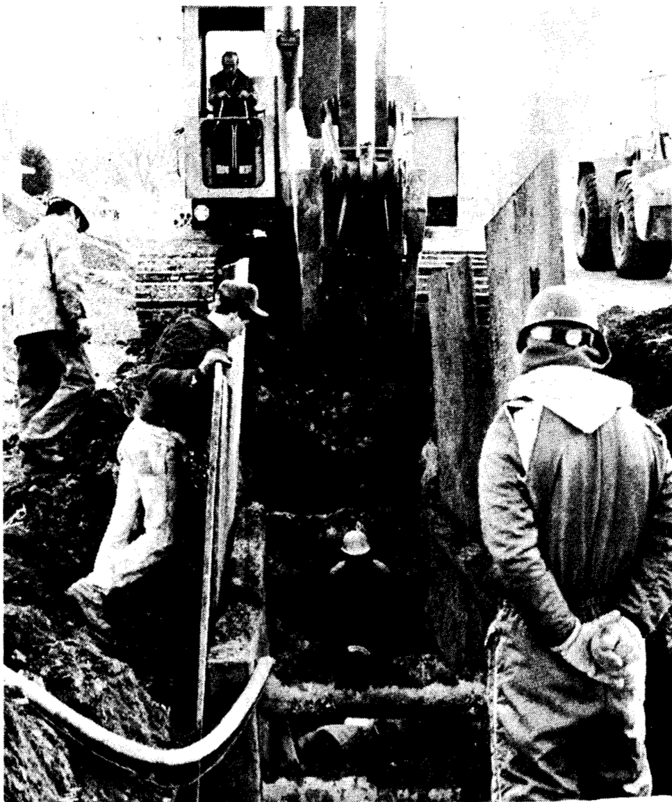
NEARING COMPLETION - The installation of the main lines of the sanitary sewer project in Gagetown is nearing completion. The lagoon and individual hookups are expected to be finished in the spring.
