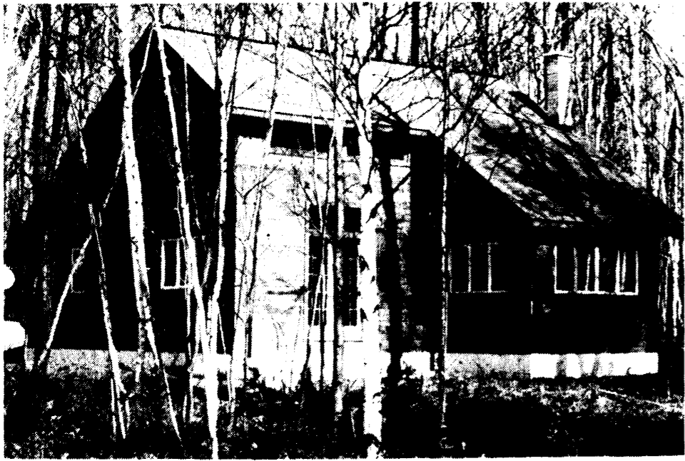
NESTLED IN the woods is the super insulated home that has been built to gain heat from the winter sun through the large glass windows on the south side of the home.
