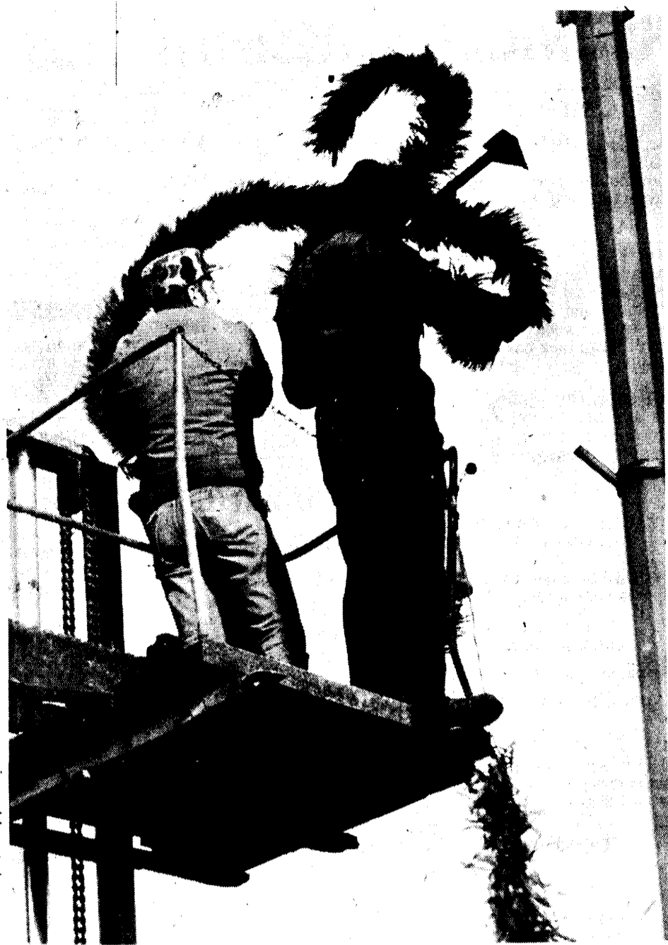
A FAMILIAR job for village workers is erecting Christmas decorations on Main Street. The work started last Wednesday.
